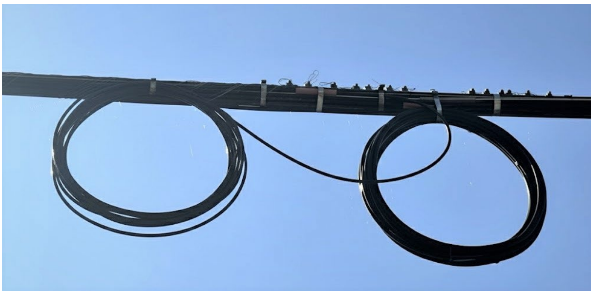
Figure 10.3 - Metallic Ties Supporting Temporary Fiber Storage
