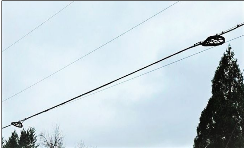
Figure 10.9- Proper Aerial Storage of Fiber Optic Cable
