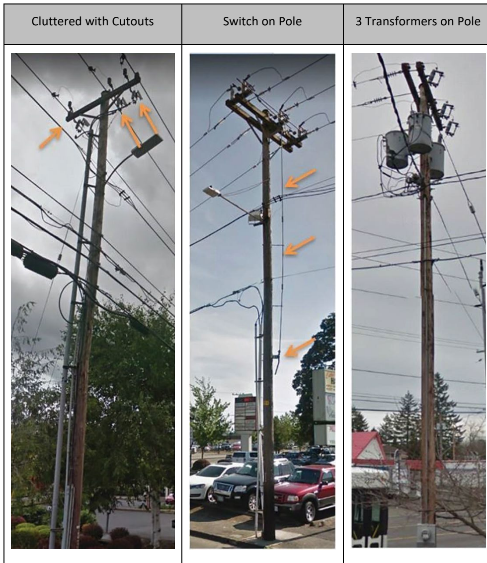
Figure 9.12 - Poles Not Suitable (Poor) for Wireless Co-Location
