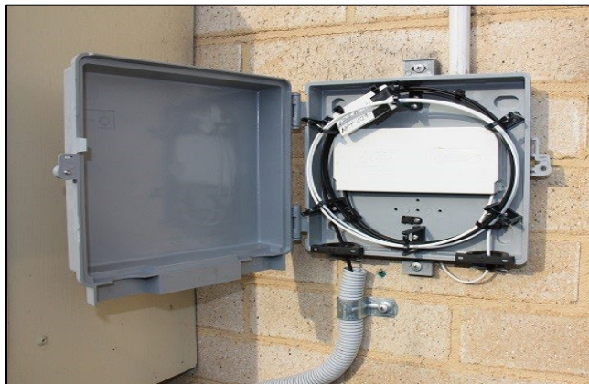
Figure 10.11 - Examples of Fiber or Cable Storage at Premise
