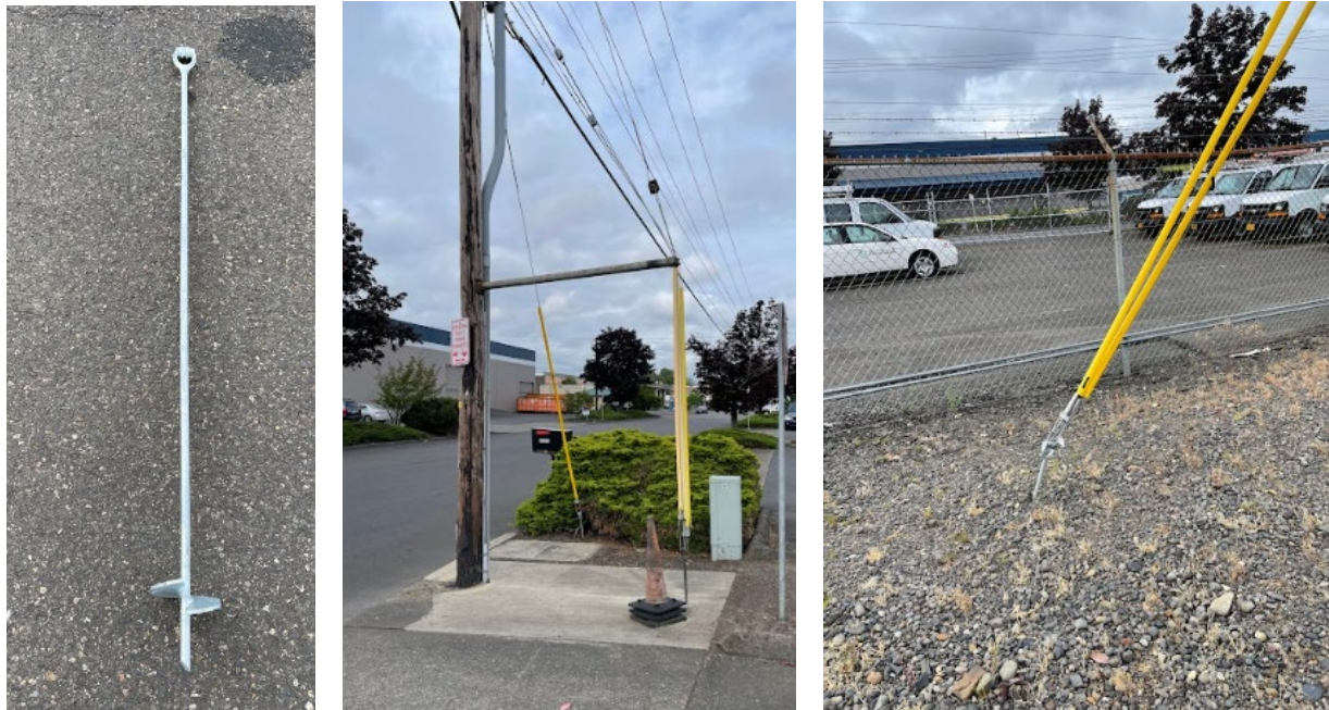
Figure 1.1 –Left-Standard Triple Eye Anchor/ Middle-Correctly Installed Sidewalk Anchor Guy & Guy Marker/ Right-Standard Anchor Guy & Guy Marker
