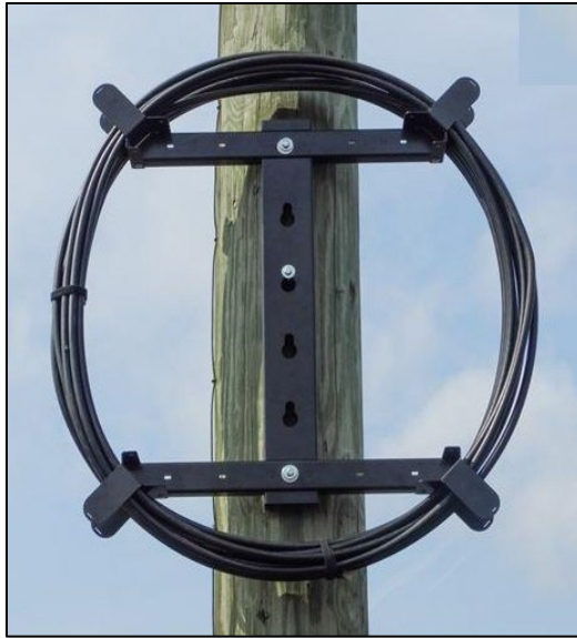
Figure 10.5 - Snowshoe-clamped, Fiber lashed
