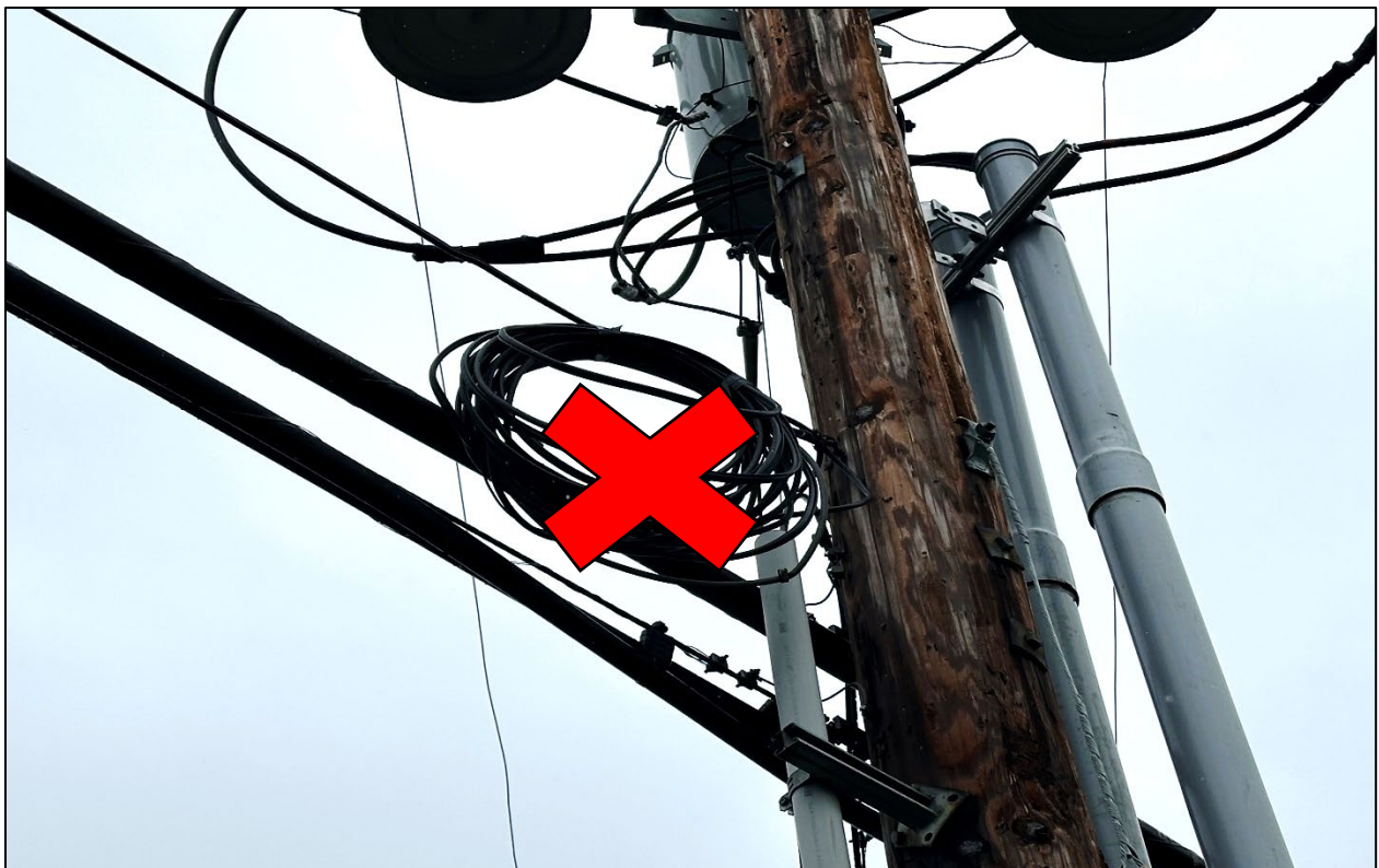
Figure 10.13 - Improper Storage of a Drop with Large Coil Tied Off with Tape Directly Next to Pole
