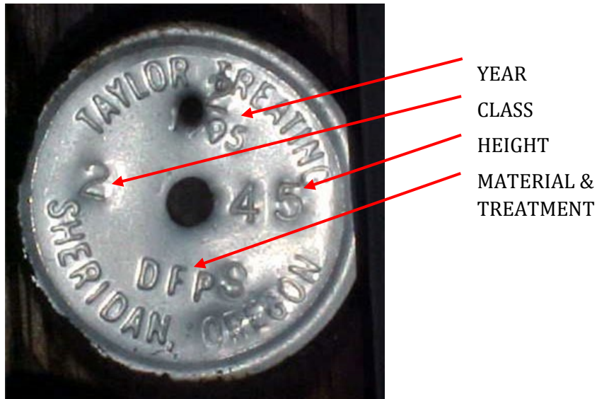
Figure 4.1 - Metal Tag Method of Identification
