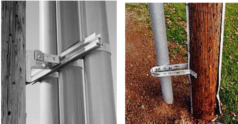
Figure 5.7 - Conduit Installation: Attachment to Standoff Brackets with Conduit Clamps
