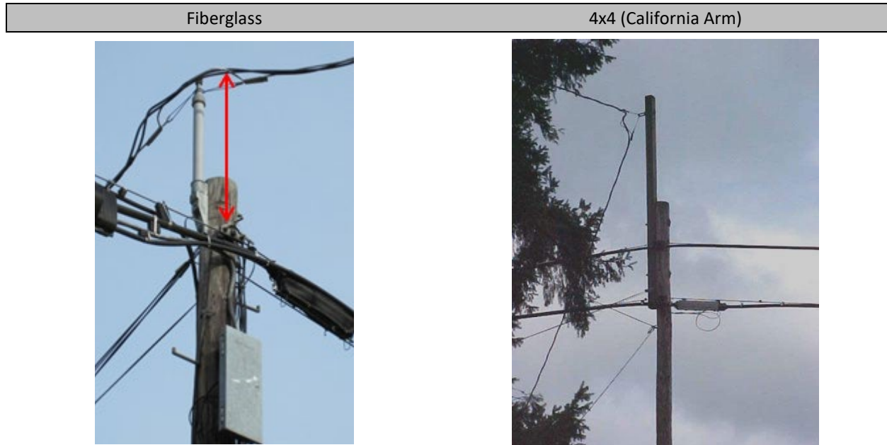
Figure 4.4 - Pole Top Extension Types
