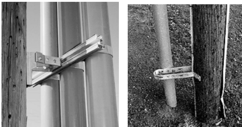
Figure 37 - Conduit Installation: Attachment to Standoff Brackets with Conduit Clamps
