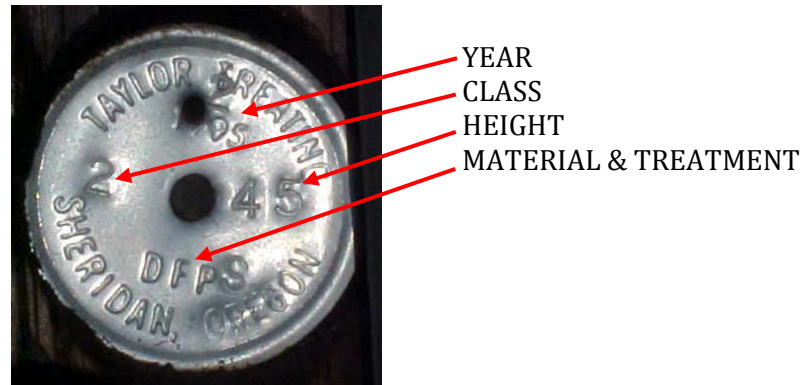
Figure 23 - Metal Tag Method of Identification
