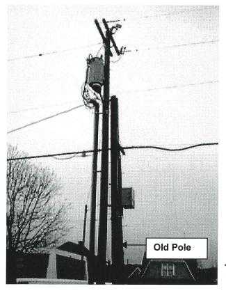
should have been completed more than a year ago. Note the new replacement pole (with transformer and crossarms) and the old pole still tied off with a rope to its right. Also, observe that a telecommunication cable and cabinet are still attached to the old pole. The installation contains violations of NESC Rules 236 (climbing space obstructed), 234.B. (inadequate cable clearances to an unattached structure) and 214.A.5. (known unsafe conditions not corrected in a prompt manner).
